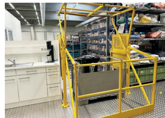
The material bin filled with granulate is lifted to the upper floor towards the central materials handling system, using a fork lift with sophisticated safety devices.
