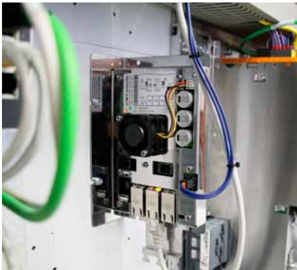
View of the router installed in the control cabinet of the injection molding machine.
