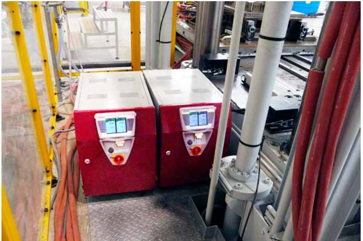
Two of the three WITTMANN TEMPRO plus D180 temperature controllers that were installed at Wethje.
